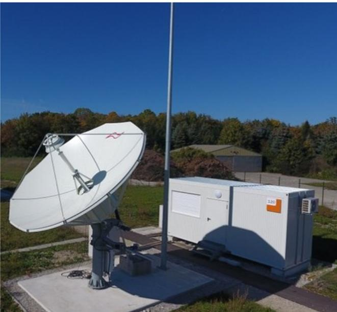
Fig. 7. GEO transmissions with a 4.9 m satellite antenna and co-located gNB and UE in the laboratory building.
